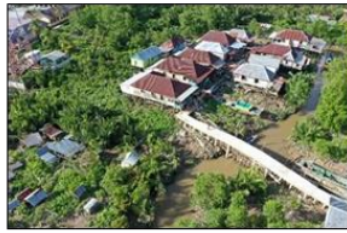
(a) Bridge of Indah Sungsang I;
